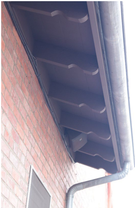
Photo 8 Wood corbels under roof eave at east elevation (November 1, 2024)
